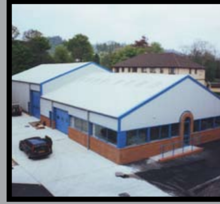
Post Advanced Roofing
