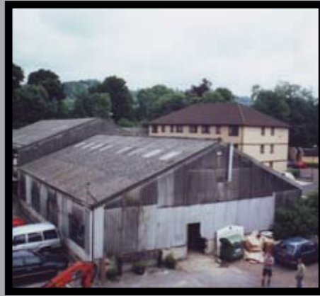
Pre Advanced Roofing
