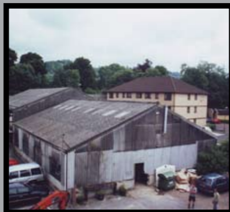
Pre Advanced Roofing
